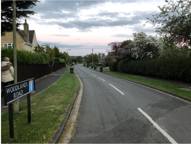
Figure 45 Woodlands Road, looking east from junction with Woodstock Road
