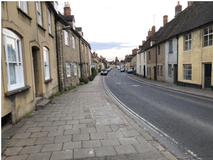
Figure 31 West End, wider footpath section, looking south-east
