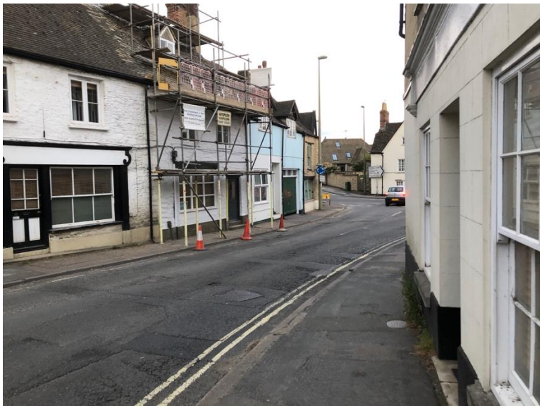
Figure 33 West End looking towards Bridge Street/Newland/Woodstock Road junction
