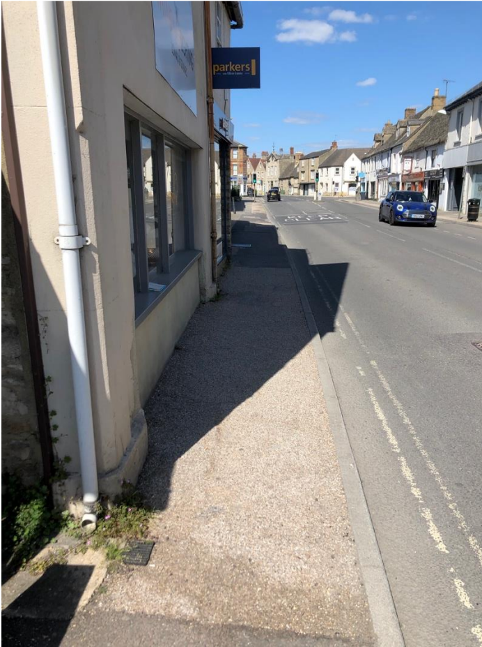
Figure 22 High Street towards north-west end junction of Witan Way
